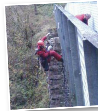
The specialist rope access team assist with the installation of the non-slip sheeting; and the finished result
