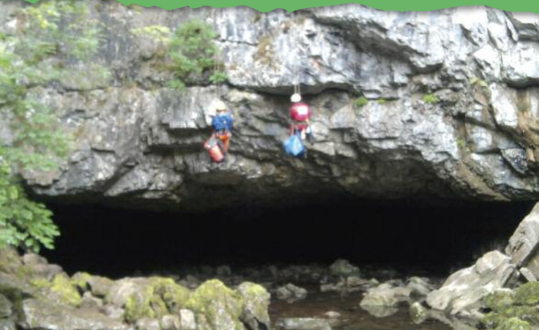
The specialist rope team inspect the cliffs above the Porth yr Ogorf cave entrance at Cwm Porth
