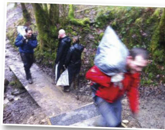
Hardworking volunteers shifting the 10 tonne of gravel for re-surfacing works.
