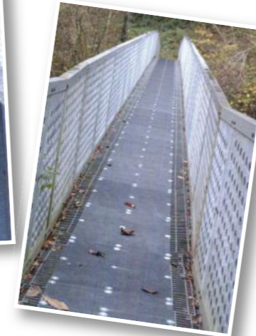
The specialist rope access team assist with the installation of the non-slip sheeting; and the finished result
